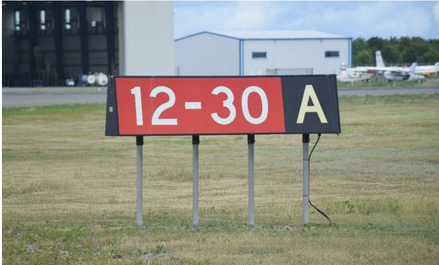
Figure 12 - Runway-Taxiway Intersection Mandatory Instruction and Location Sign
