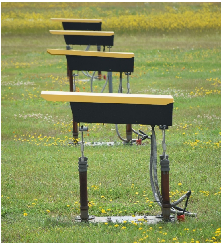
Figure 38 - Precision Approach Path Indicator (PAPI) Side View
