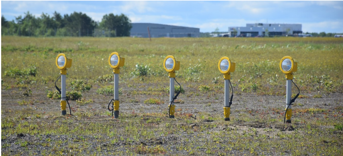
Figure 42 - Short Simplified Approach Lighting with Runway Alignment Indicator Lights (SSALR) Row of White Lights
