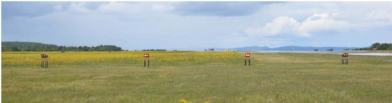
Figure 38 - Precision Approach Path Indicator (PAPI) Side View
