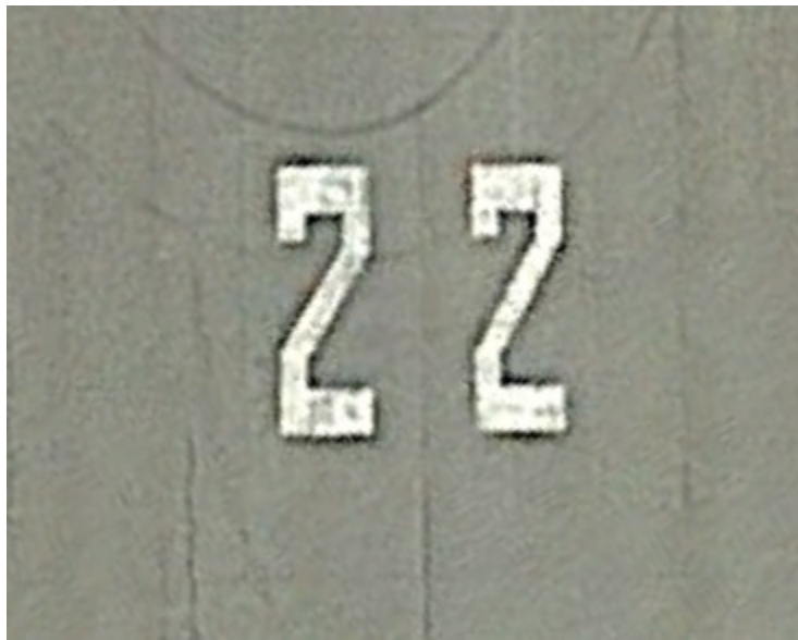
Figure 18 - Runway Designation Marking
