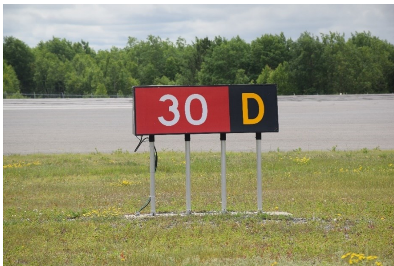
Figure 13 - Runway-Taxiway Intersection Mandatory Instruction Sign Located at a Runway Threshold
