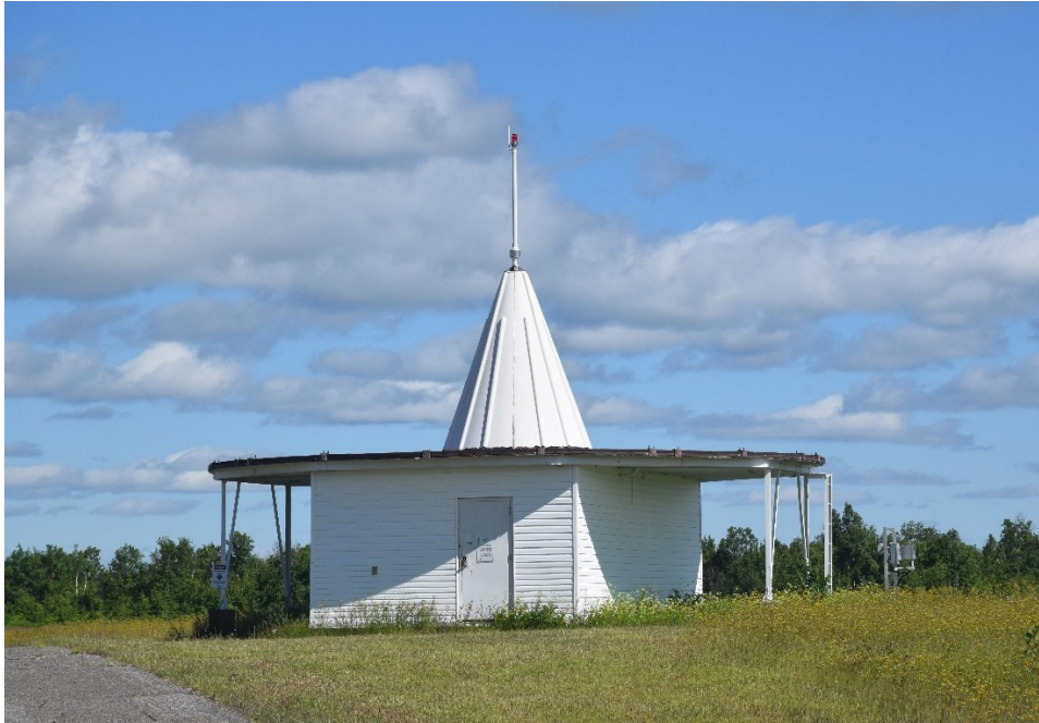
Figure 47 - VHF Omnidirectional Range (VOR)
