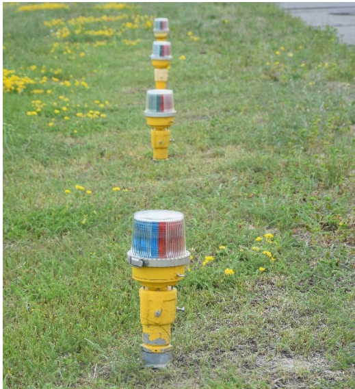
Figure 24 - Runway end and Threshold Lights on Runways 04, 12 and 30 Diagram
