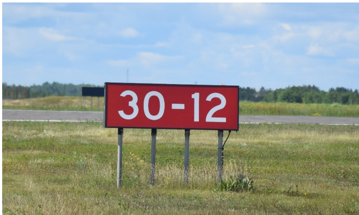
Figure 11 - Runway-Runway Intersection Mandatory Instruction Sign
